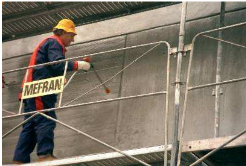
Photo 4.5: Application of inhibitor
