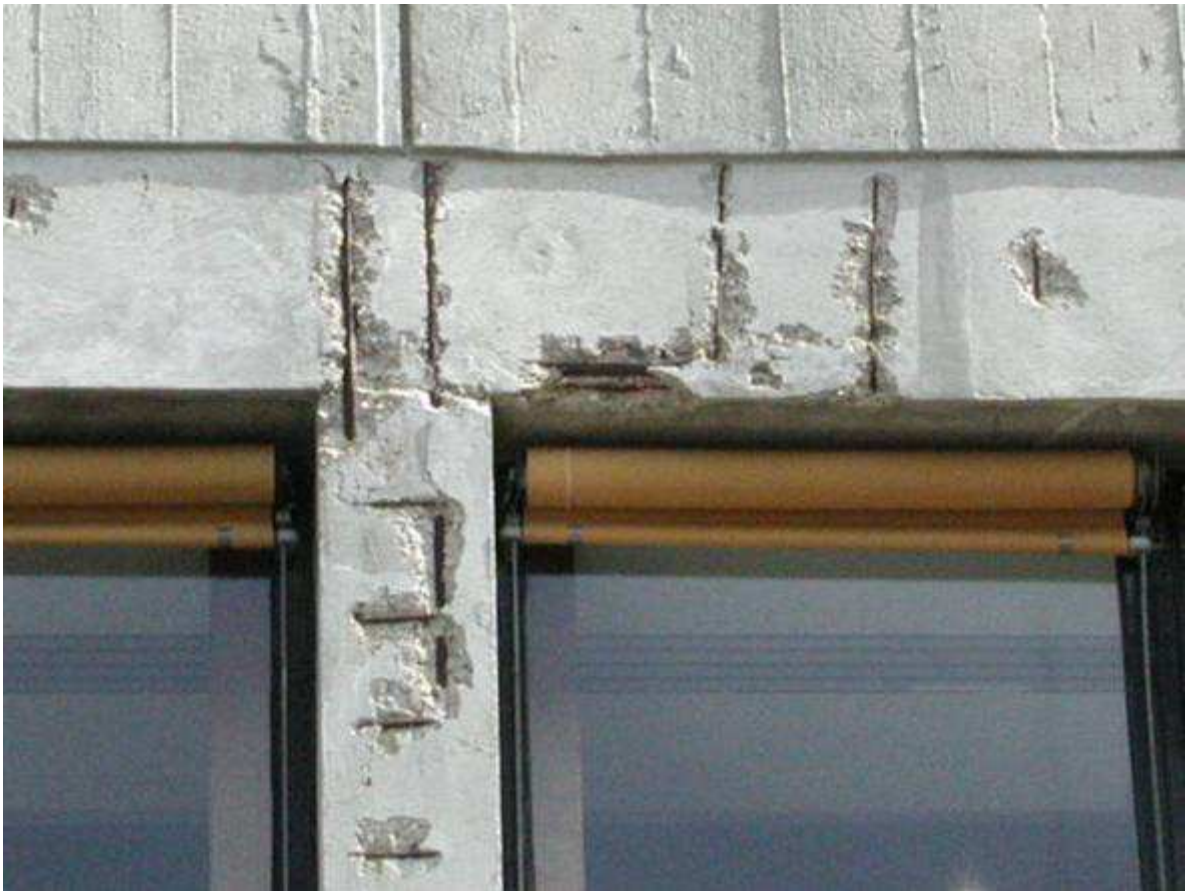
Photo 1.1: Spalls on a facade
