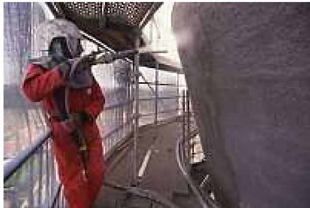
Photo 3.2: Spraying concrete under hard conditions
