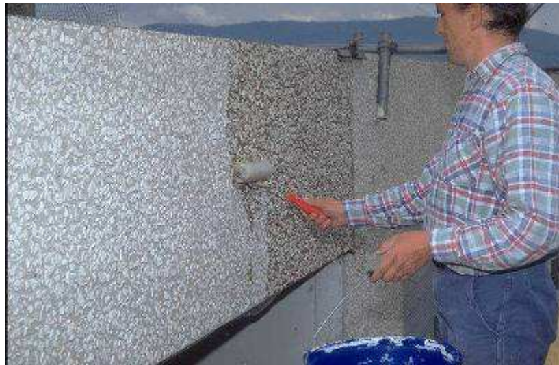
Photo 4.4: Application of inhibitor
