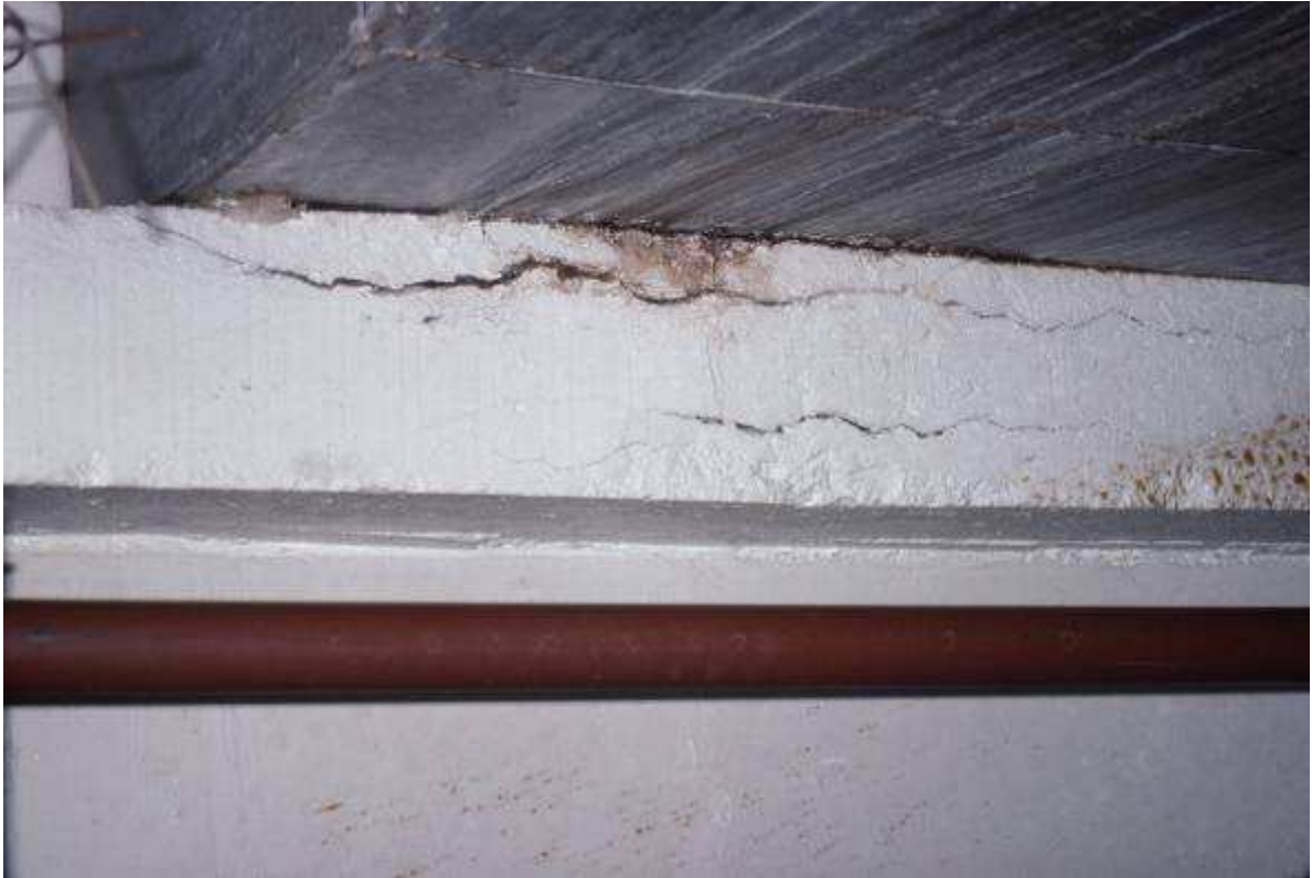
Photo 1.2: Corroded beam supporting a reservoir
