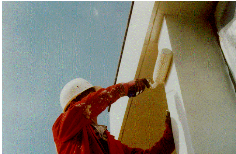
Photo 4.6: Application of inhibitor
