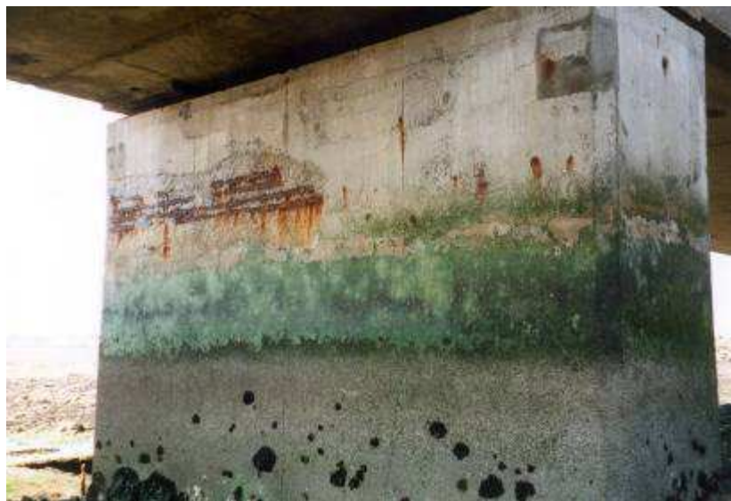
Photo 1.7: Bridge piling in a tidal zone
