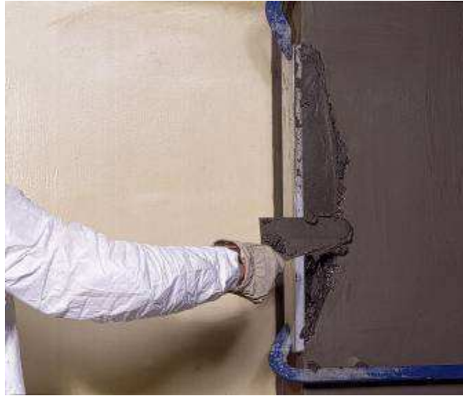
Photo 4.2: Replacing concrete cover
