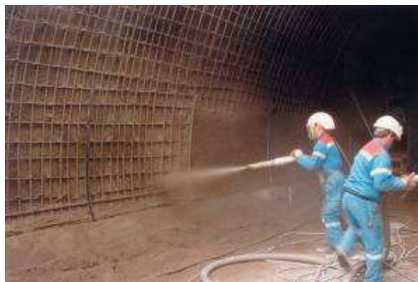
Photo 4.7: Projection of concrete
