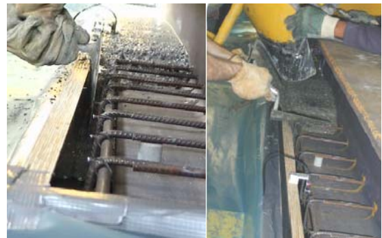
Figure 3 : Casting of the beam at LCPC Coulage de la poutre au LCPC
