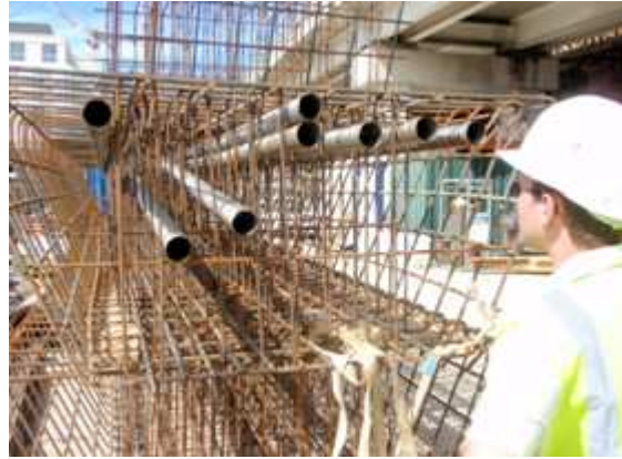
Figure 19: Ferrailage des nervures
