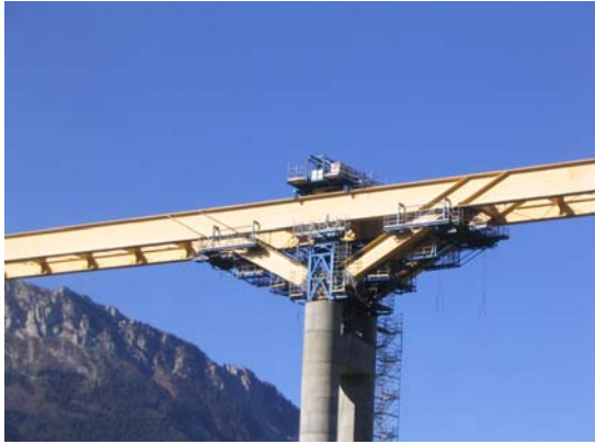
Bracon positionné entre le tablier et la pile Metallic support located between the deck and one pier
