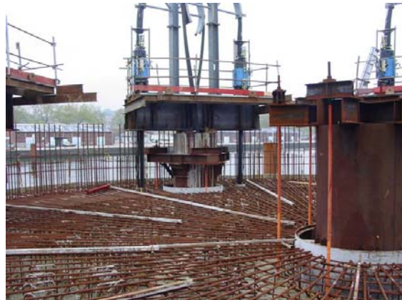
Photo 7: VSL jacks: 330 tonnes each Vérins de descente VSL : 330 T unitaire
