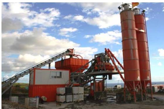
Photo 2 : Centrale à béton sur le site Concrete batching and mixing plant on the site
