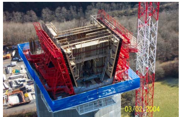
Once the lower block was complete, the forms for the webs of the pier segments were put in place; this visibly complex operation was reexamined in great depth during the design stage to improve the progression of the phases.
