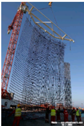
Fig 16 : Levage cage armatures / Reinforcement grid erection
