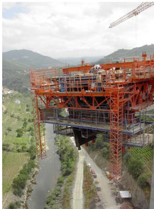
Photo 5: Travelling form Equipage mobile de bétonnage
