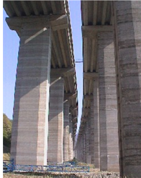
Fig 1. View from the ground at the highest piers location
