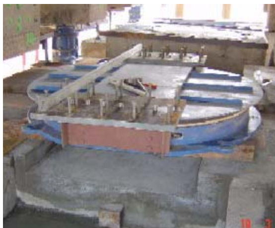
Fig. 11. New bearing device for intermediate diaphragms
