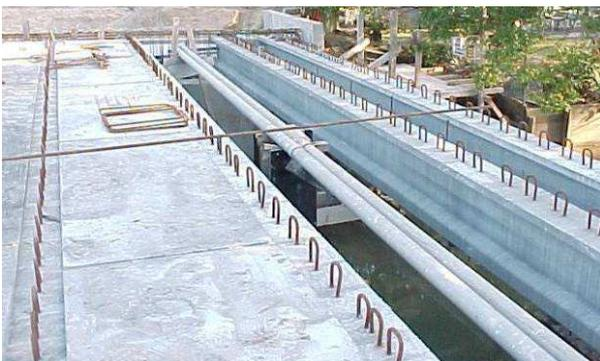
b. Installed beams and formwork slabs
