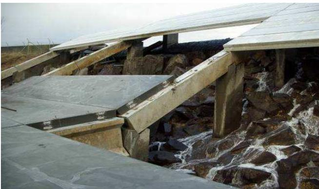
(c) Installation of new UHPC panels
