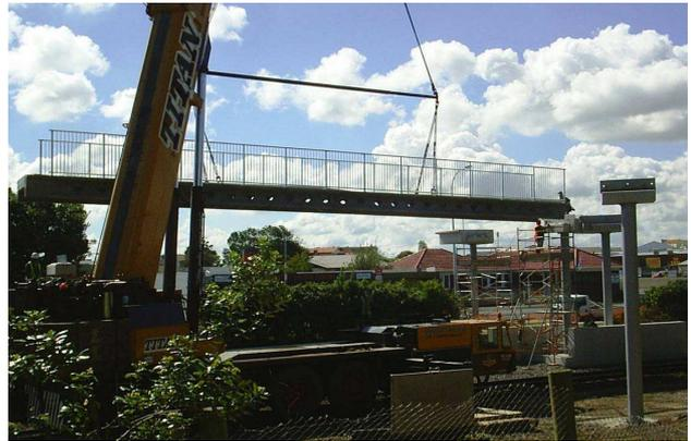
e. Lifting a UHPC span (with hand railing attached)
