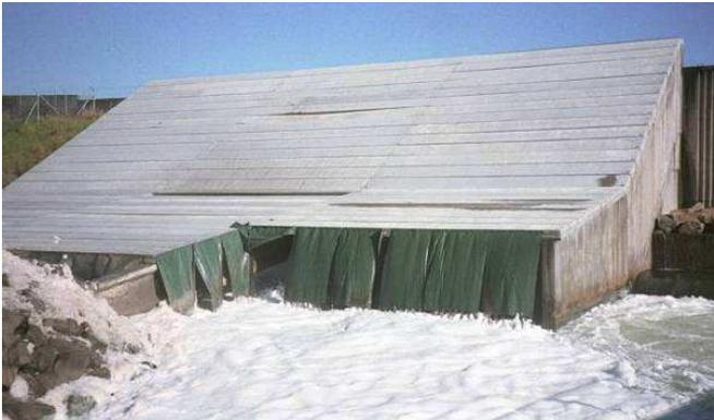
(a) Weir prior to upgrade showing failed planks
