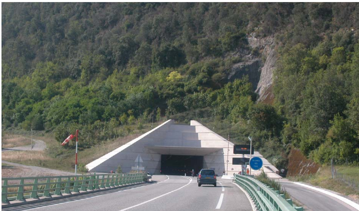
Tête nord – Vue générale / Northern portal – General view
