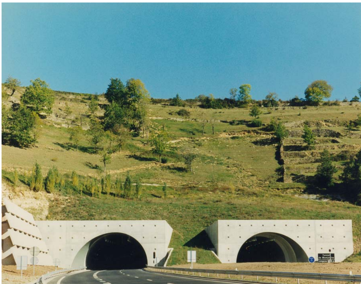
Tête sud / Southern portal
