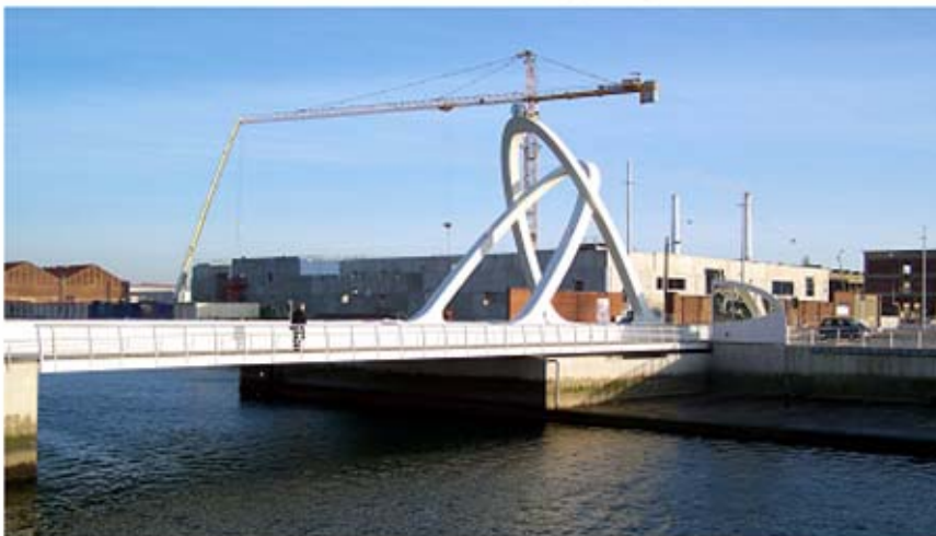
Le Havre – Vatine swing Bridge
