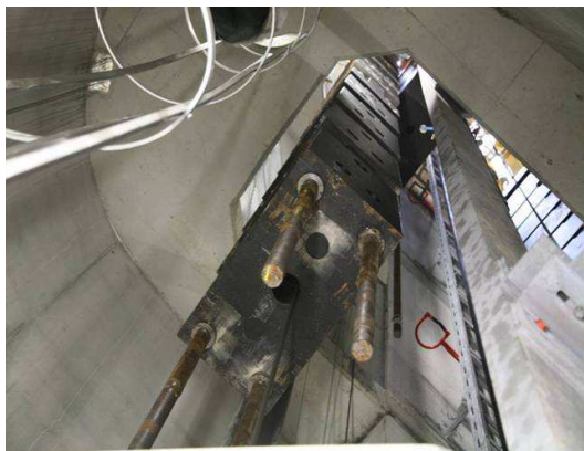
Assemblage des contrepoids
