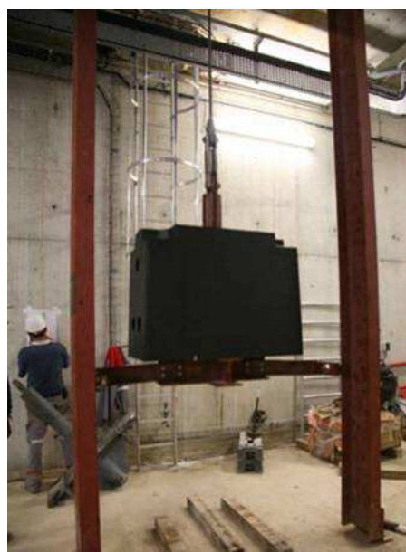
Levage des contrepoids
