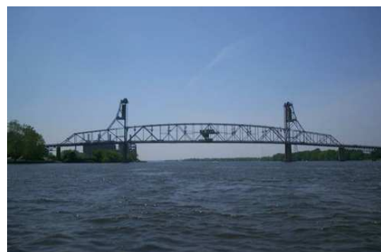
Burlington - Bristol - Pennsylvania (travée de 164 m)
