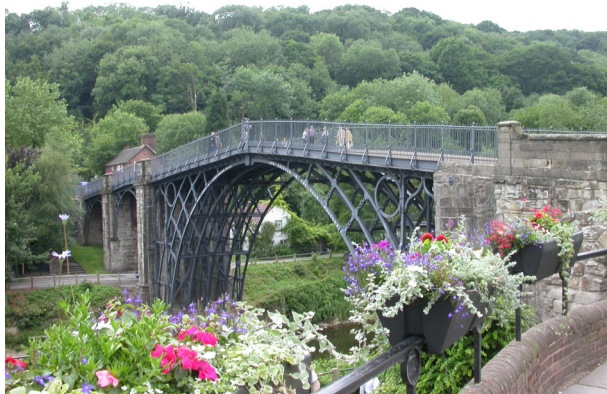
Figure 11 : Iron Bridge – Birmingham (1779)
