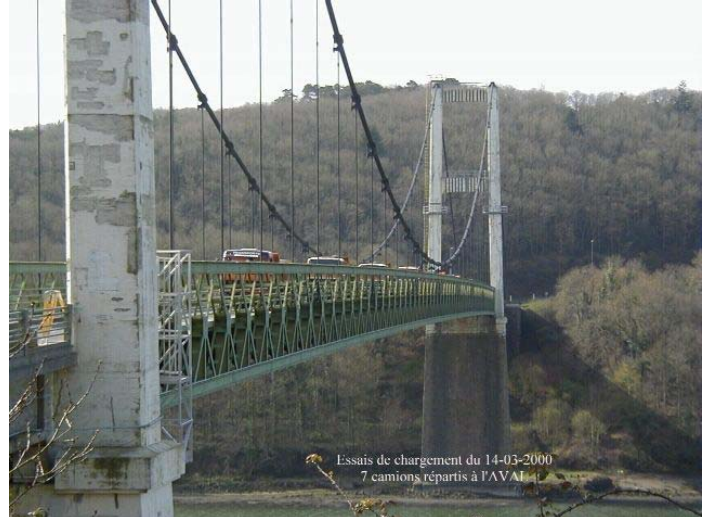
Figure 21 Le pont suspendu
