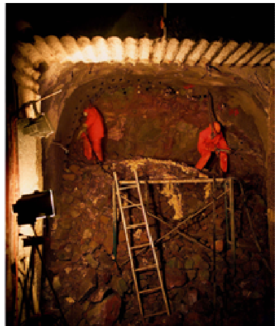
Photo 4 – LMC Tunnel - excavation of frozen ground / excavation du cross-passage
