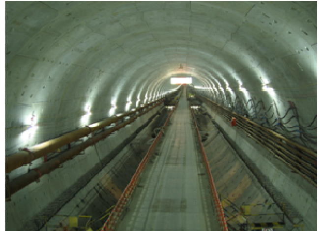
Photo 10 – Chong Mingtunnel – TBM cutter head and Tunnel under construction
