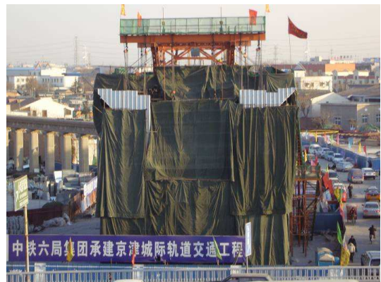
Figure 20 – Pier cast under heated enclosure
