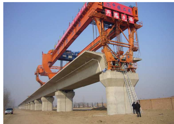
Figure 13 - Launching gantry
