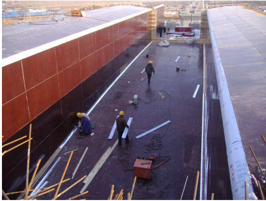
Figure 16 - Préparation du coffrage Preparation of formwork
