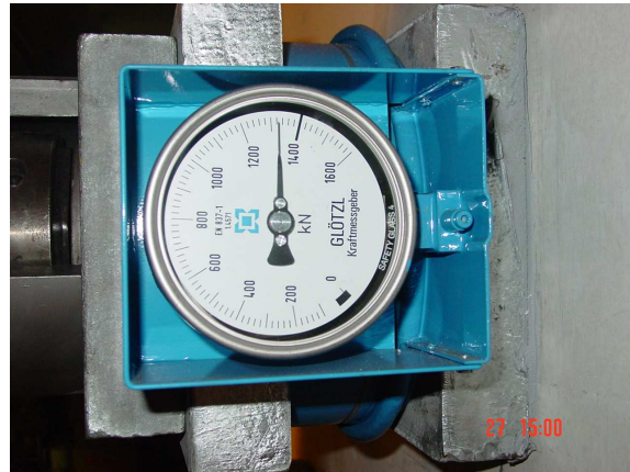
Photo 19: 3 or 4 short bars on each blister are equipped with load cells so the residual tension can be read directly in kN.
