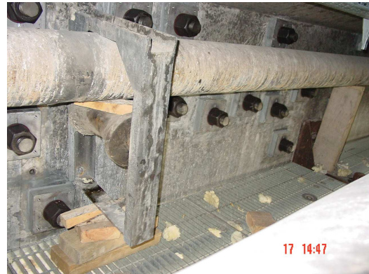
Photo 17: The presence of utilities placed considerable restrictions on where the reinforcements could be placed. During drilling, the gas pipe was protected with plywood.
