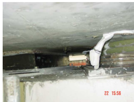
Photo 26: A sand box, flat jacks, distribution pads and sliding plate can be seen in view of jacking and unjacking of the deck.
