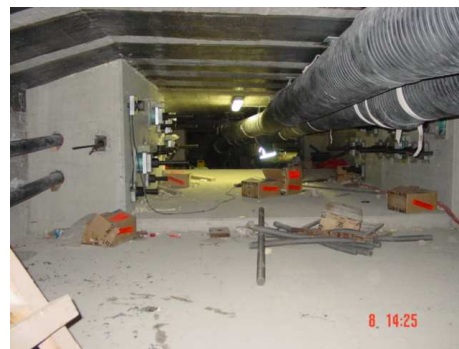
Photo 21 : Reinforcement of top slab with TFC® carbon-fibre bonded composite to transfer distribution stresses from additional cables.
