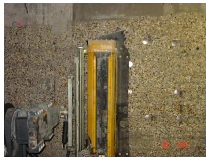
Photo 15: Remote controlled high pressure water spraying of concrete surfaces at 200 MPa. Demountability of the tool enabled it to pass through a 1.20 m x 0.80 m manhole in the girders.
