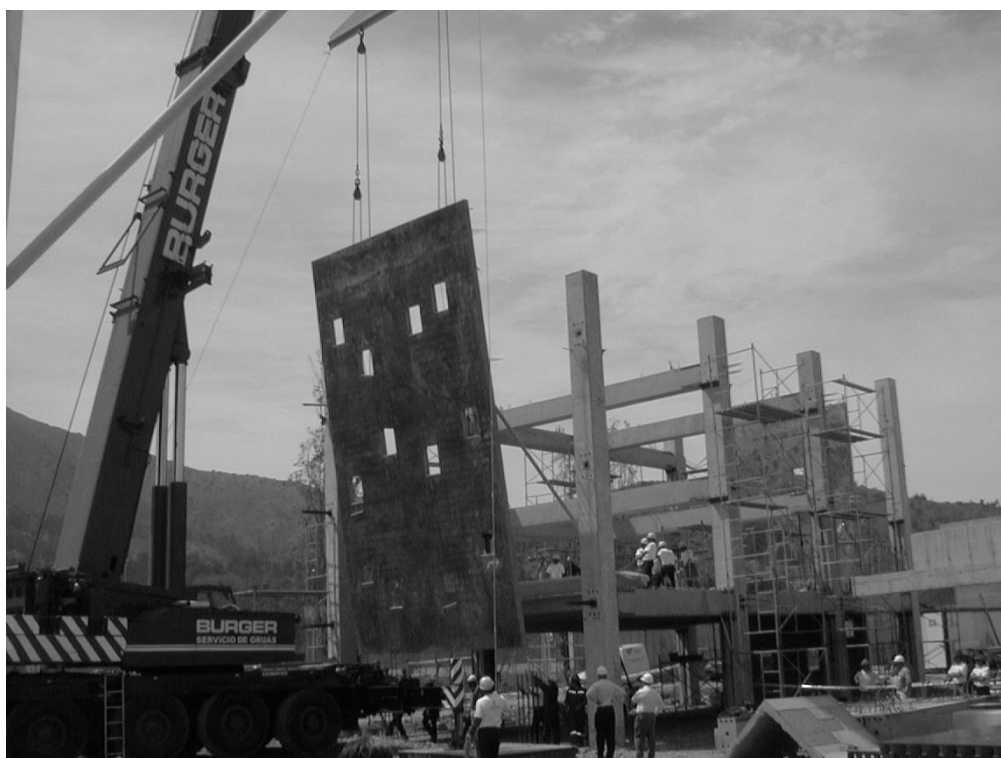
Fig. 5-53: Erection of a cantilever wall in a building in Chile built with hybrid frames and walls (Courtesy of P. Bonelli)
