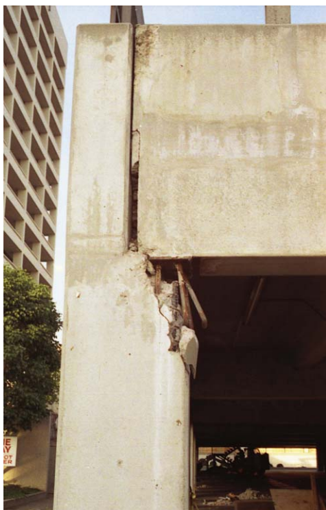
Fig. 2-17: Brittle failure of beam-column pin connection at top of corner column (1994 Northridge earthquake)
