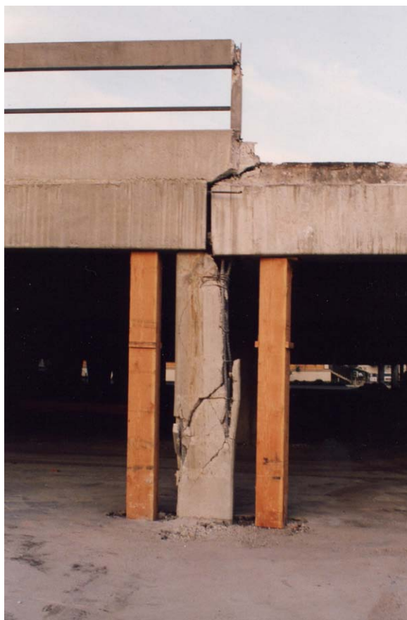
Fig. 2-16: Beam-to-column connection failure and shear failure of column in precast concrete parking structure (1994 Northridge earthquake)
