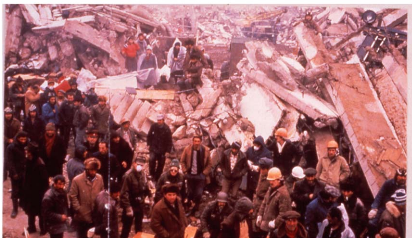
Fig. 2-2: Collapse of precast buildings in Leninakan, Armenia in 1988 [EERI (1989
