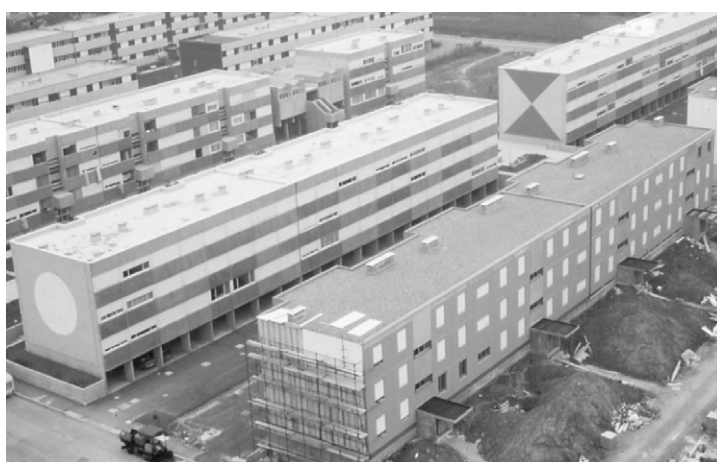
Fig. 5-49: Example of a large residential complex in Italy built using large panel construction (Courtesy of M. Menegotto)
