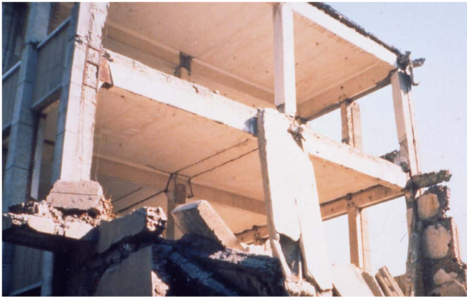
Fig. 2-12: Failure of a poorly detailed beam-column connection (1976 Tangshan earthquake, China)
