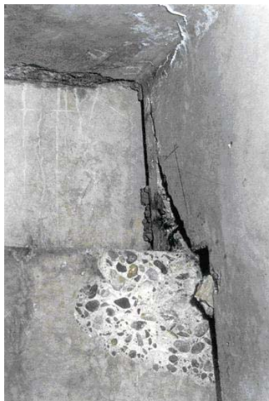
Fig. 3-8: Double tee, stepped end detail, that has been damaged by thermal bowing in a parking building
