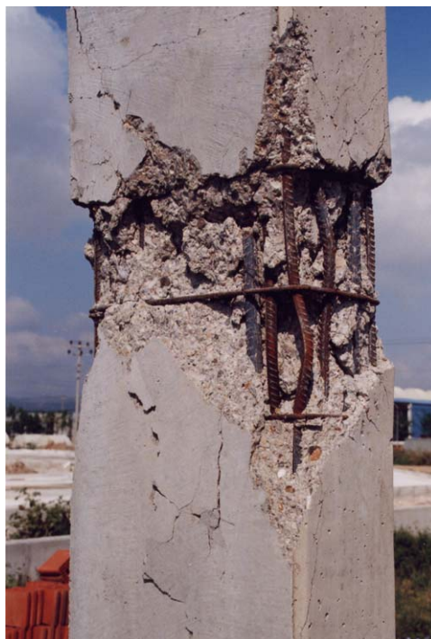
Fig. 2-8: Close-up of poor column details (1999 Kocaeli earthquake)
