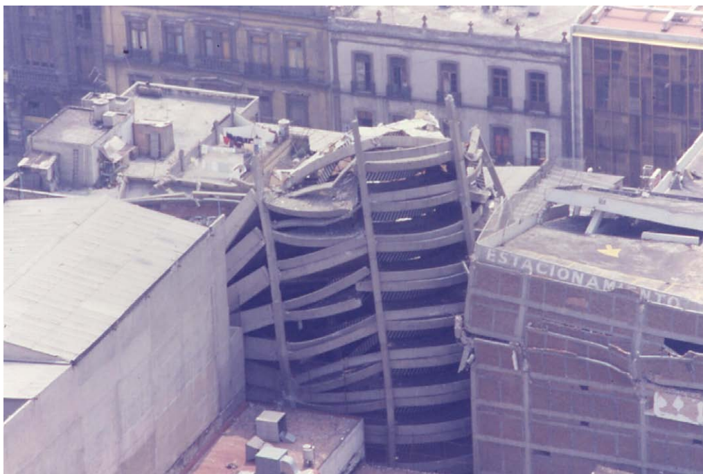
Fig. 2-21: Collapse of precast concrete parking structure due to pounding against adjacent structure in Mexico City (1985 Michoacán earthquake)
