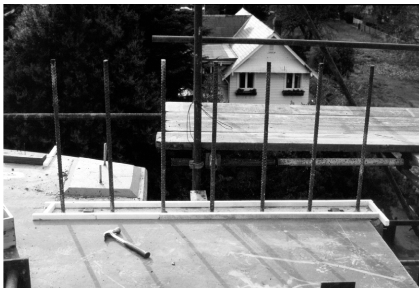
(c) Close up of horizontal connection detail
