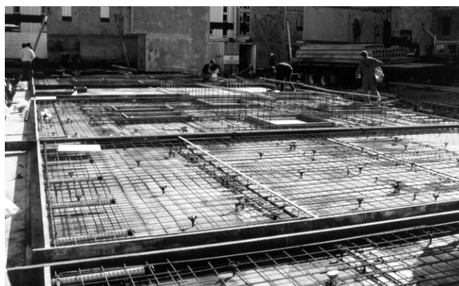
Fig. 5-51: Wall panels incorporating a connection details through grouted ducts under construction in New Zealand (Courtesy of J. Restrepo)
