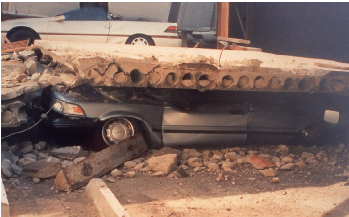
Fig. 2-9: Collapse of precast concrete hollow core floor (1994 Northridge earthquake)
