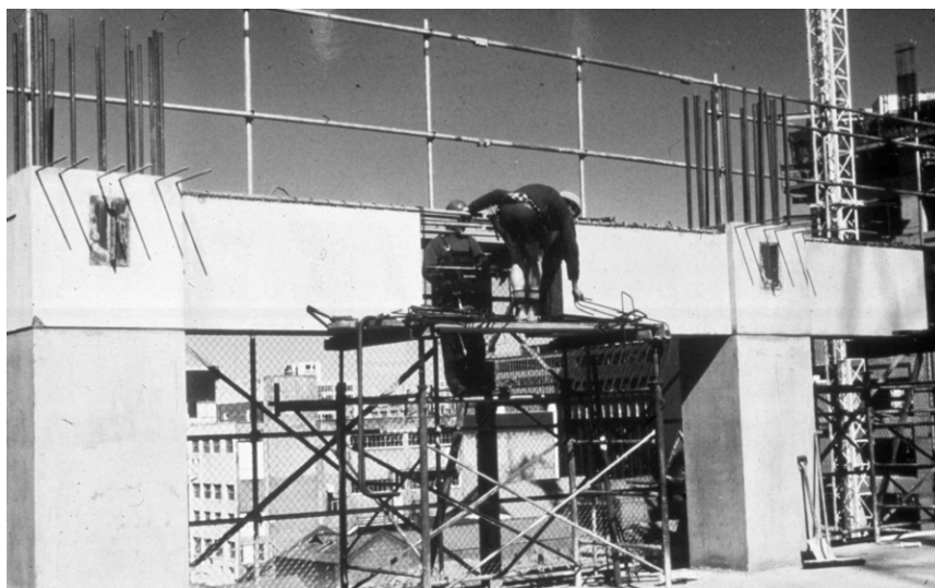
Fig. 5-26: Example of a connection with double-straight bar laps in a building in New Zealand (Courtesy of J. Restrepo)
