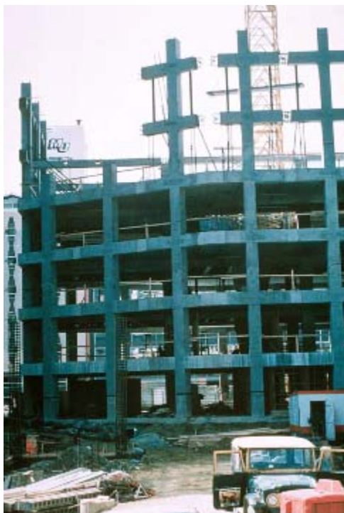
Fig. 3-4: Two storey precast beam-column units forming a perimeter ductile moment resisting frame
