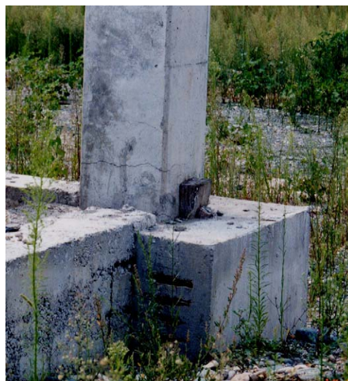
Fig. 8-4: Undamaged socket foundation (Kocaeli earthquake, Turkey 1999)
