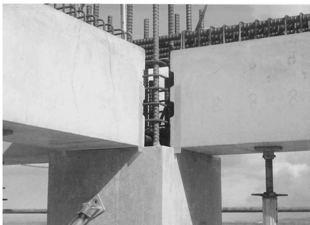
(a) Example from Japan: View of beams before the placement of the floor slab (Courtesy of F. Watanabe)
