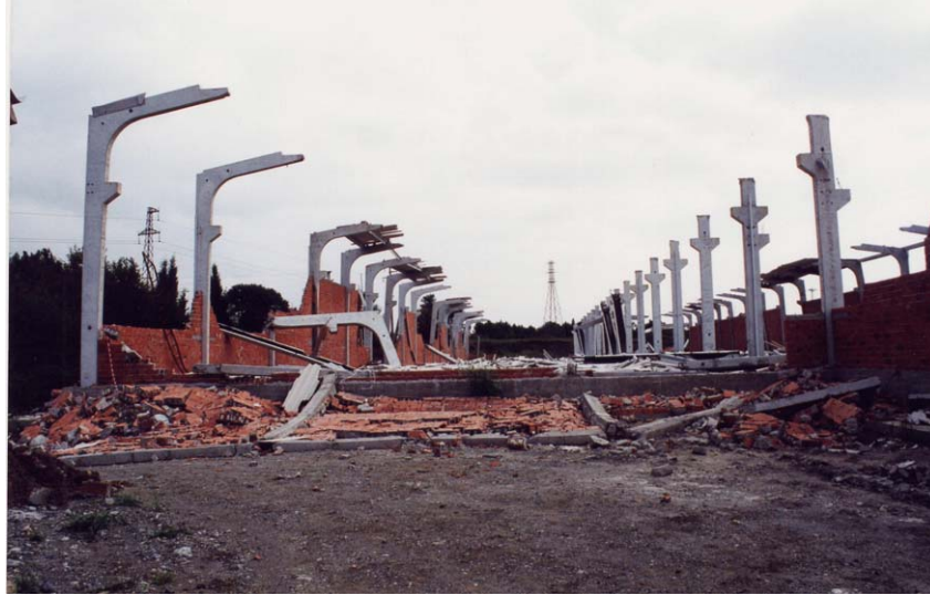
Fig. 2-19: Failure of columns due to interaction with stiff masonry infill (1999 Kocaeli earthquake)
