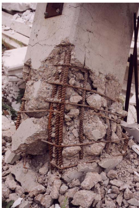
Fig. 2-5: Shear failure at base of precast concrete column (1999 Kocaeli earthquake)
