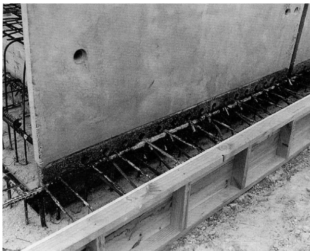
Fig. 5-45: Example of a wall embedded in the foundation beam
