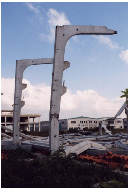
Fig. 2.7: Severe distress in precast concrete column (1999 Kocaeli earthquake)
