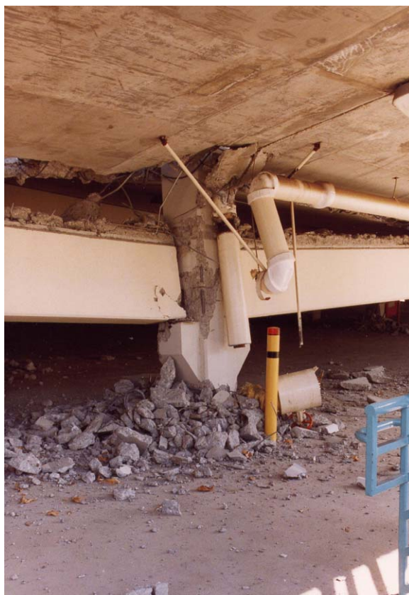
Fig. 2-3: Failure of poorly detailed precast concrete column in the 1994 Northridge earthquake
