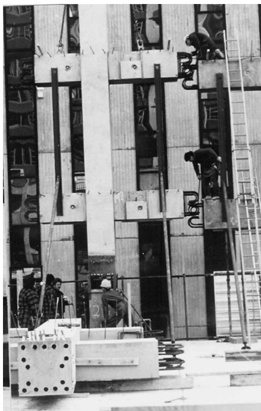
Fig. 5-34: Example of column-to-column connection through grouted steel sleeves in a building in New Zealand (Courtesy of A. O'Leary)
