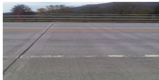
Figure 9: Otego Creek Bridge, Oneonta, NY, USA (Photo 2012)
