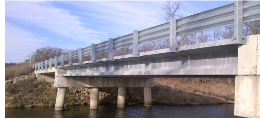
Figure 7: UHPC Pi-Girders, Jakway Park Bridge Buchanan County, Iowa, USA (Photo 2012)
