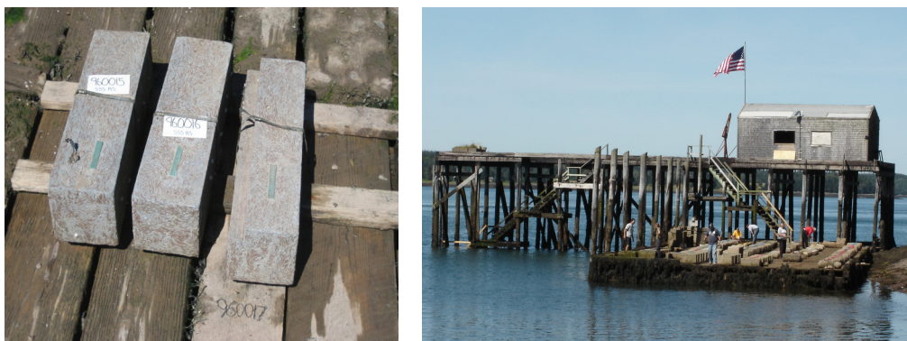
Figure 2: UHPC Prism at US Army Corps Long-Term Exposure Site, Treat Island, Maine, USA
