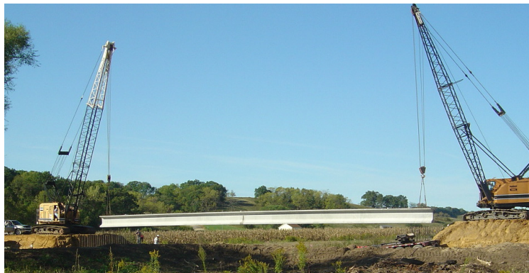
Figure 3: Placing a 34m UHPC I-Girder -Mars Hill Bridge, Wapello County, Iowa, USA
