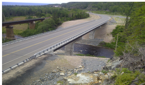
Figure 10: Steel River Bridge, Terrace Bay, Ontario, Canada (Photo 2012)
