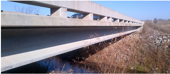
Figure 6: Mars Hill Bridge: View along UHPC I-Girder (Photo 2012)
