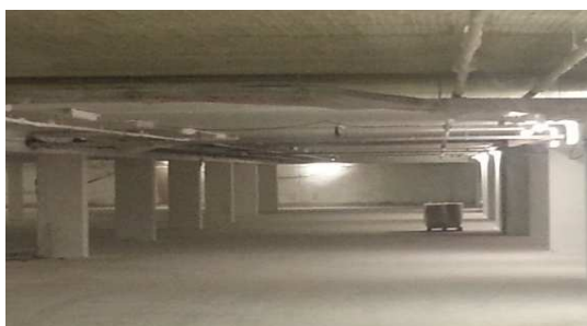
Figure 41 : Le parking enterré
