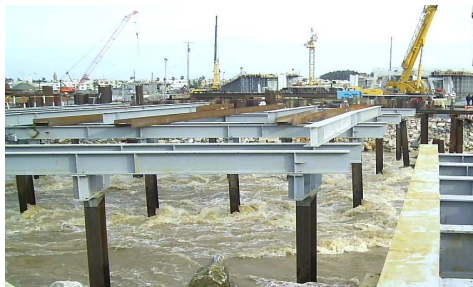
Fig. 23. Pont provisoire en construction / Temporary bridge under construction
