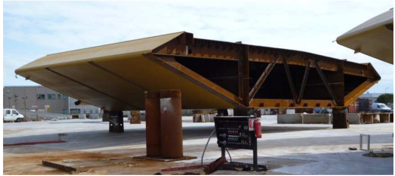
Section of the lift span box girder during manufacture
