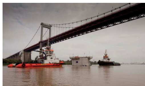
The concrete box girders during construction in the dry dock/Transport of an island under the Aquitaine Bridge
