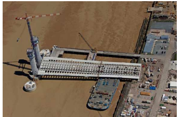
Laying of the right-bank access spans in August 2011
