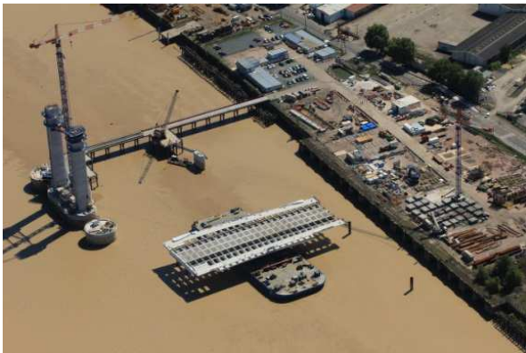
Laying of the right-bank access spans in August 2011
