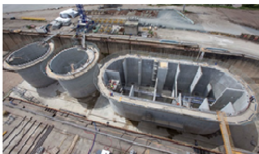
The concrete box girders during construction in the dry dock/Transport of an island under the Aquitaine Bridge
