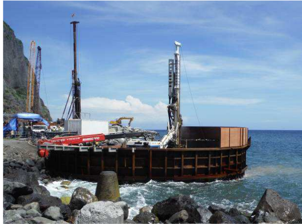
Figure 5 : View of the cofferdam
