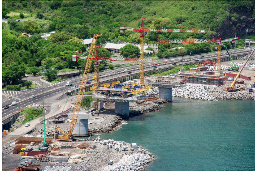
Figure 2 : General view of the viaduct under construction
