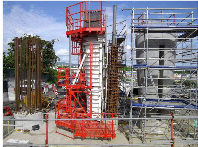
Figure 8: Pier formwork
