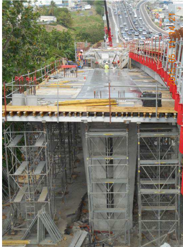
Figure 13 : scaffolding on a span
