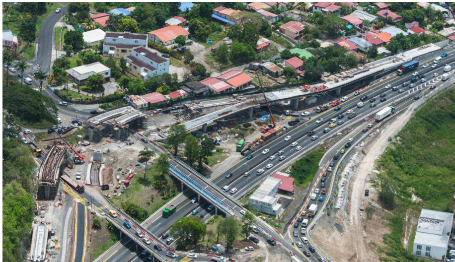
Figure 1 : General view of the viaduct under construction, May 2015
