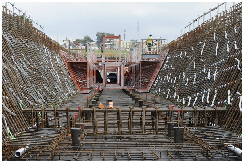
Fig.9. Internal formwork of the segments ©photothèque BYTP
