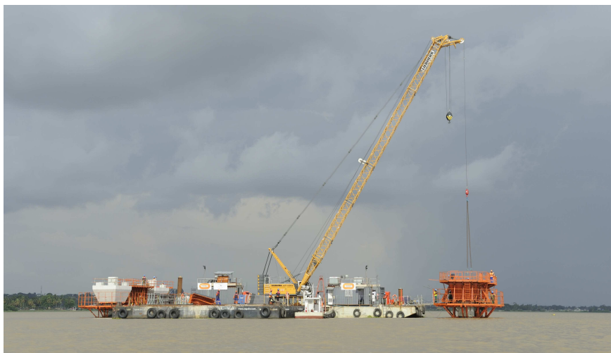
Fig.6. Formwork for a crosshead beam ©photothèque BYTP
