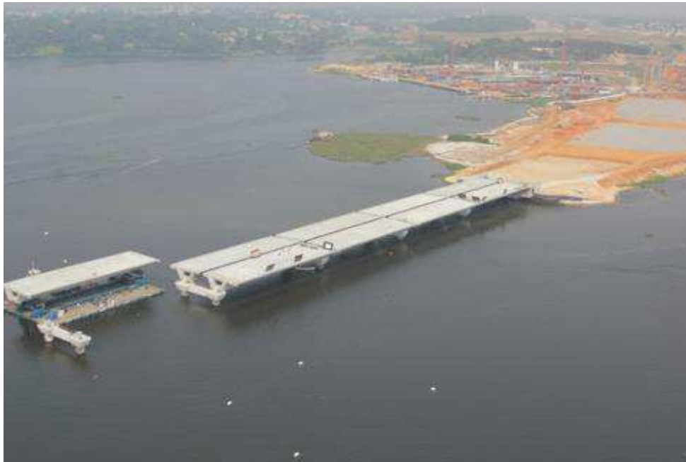
Fig.10. Placing a box girder ©photothèque BYTP
