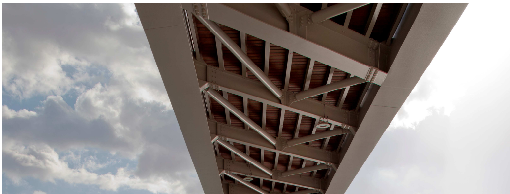
Fig.12: Below view of the deck
