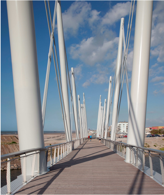
Fig.8 : View of the masts from the decks
