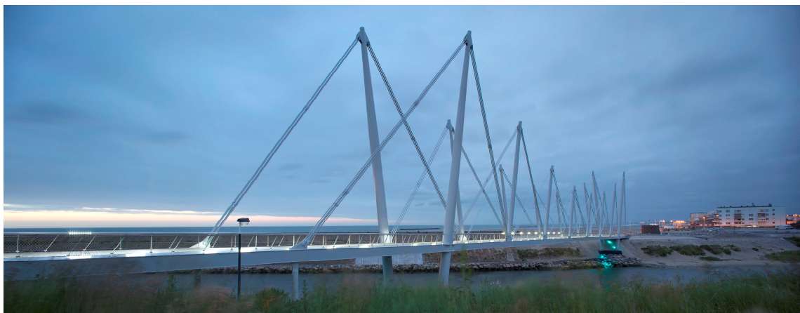
Fig. 2: View of the footbridge from the mound
