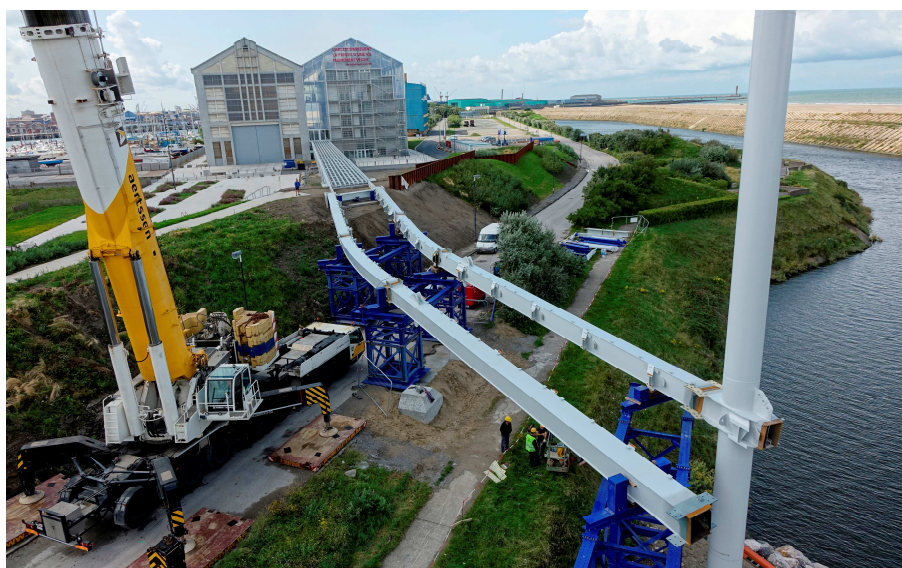
Fig 17: Assembly of the box-girders
