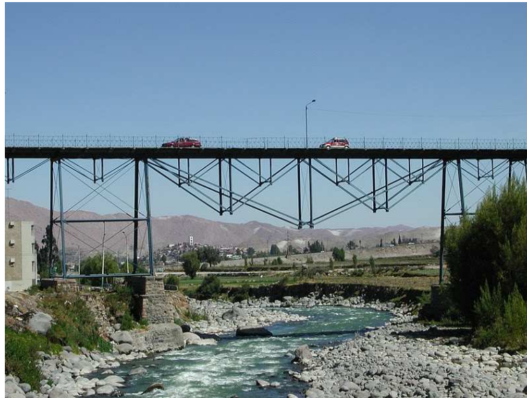
Fig.3: Bolivar Bridge in Arequipa, Peru– 1882- designed by Gustave Eiffel
