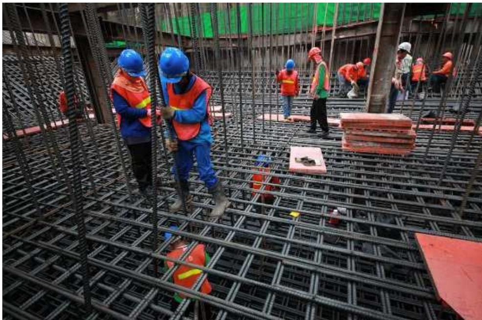
Fig.3. Reinforcement work of MahaNakhon mat foundation. (Source image courtesy of PACE Development PLC)
