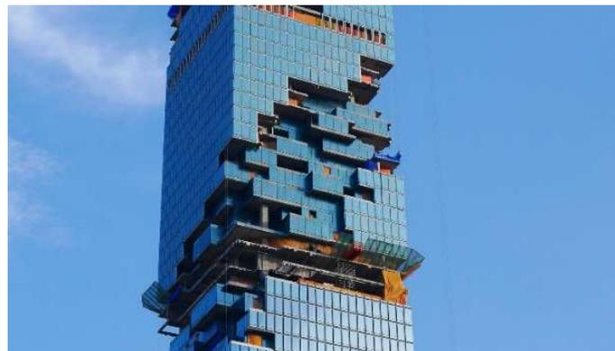
Fig.10. Pixelation of MahaNakhon tower. (Source image courtesy of PACE Development PLC)
