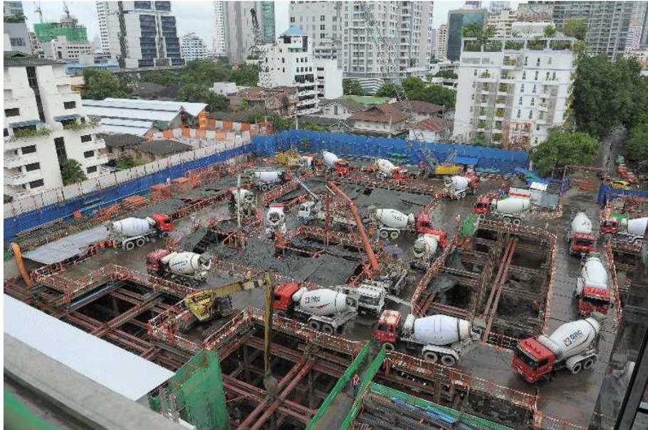
Fig.6. Concrete trucks on the mat foundation casting date. (Source Bouygues-Thai)
