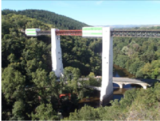
Figure 12: Scaffolding on the Rouzat viaduct
