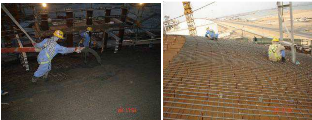
Figures 22: pouring of the dome roof
