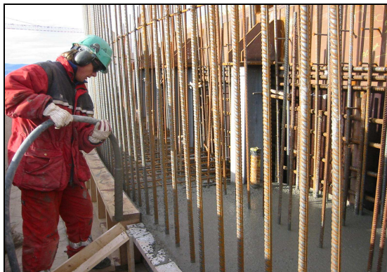
Figure 18: pouring of the wall top part
