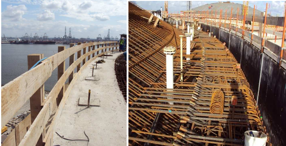
Figures 20: pouring of end of wall and roof beginning
