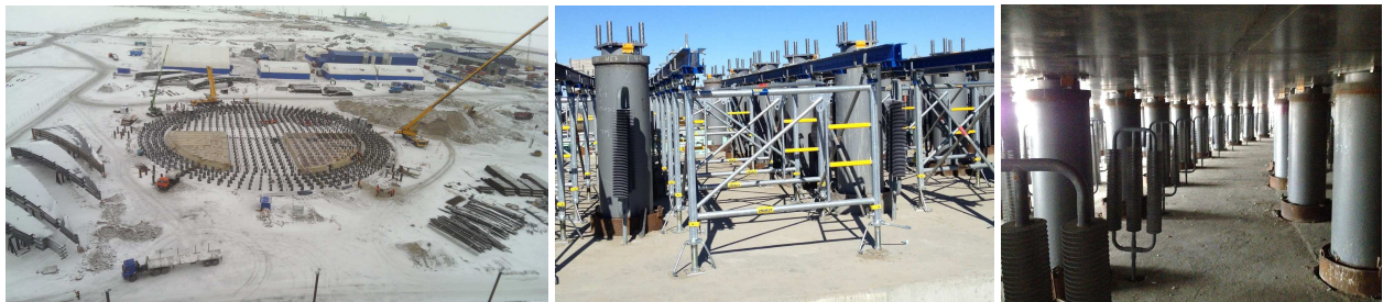
Figures 14: heat-stabilizers, the slab and the elevated raft
