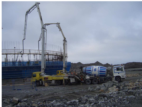
Figure 15: raising of the formwork
