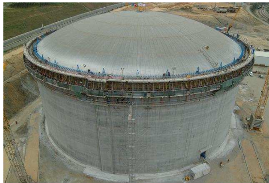
Figure 19: the steel roof liner before pouring
