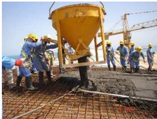
Figure 21: pouring of the roof outer ring phase
