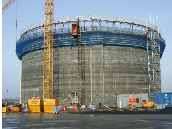
Figure 16: slipform operations
