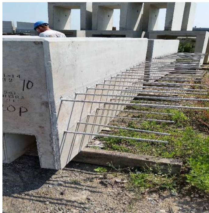
Figure 9. Precast coping used as a top out
