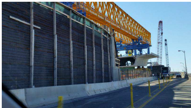
Figure 3. Temporary Terratrel wire facing for Phase 1
