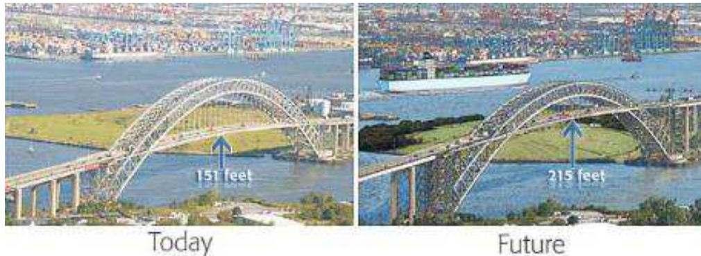
Figure 10. Raising of the Bayonne Bridge
