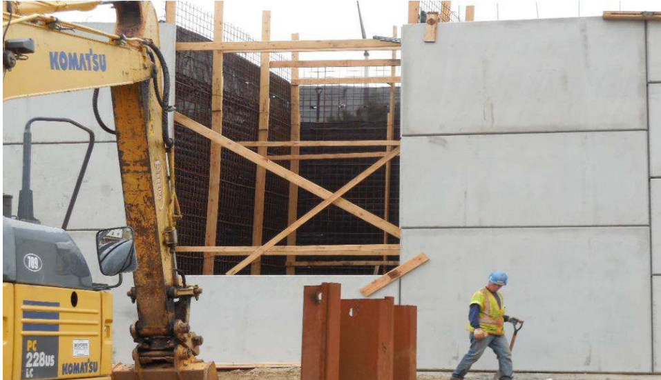
Figure 8. Terratrel “blockout” to install Reinforced Earth
