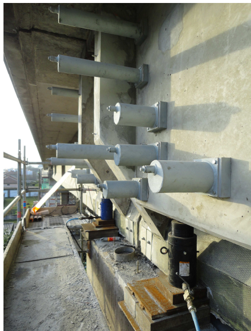
Figure 8: concrete anchorage block at beam extremity
