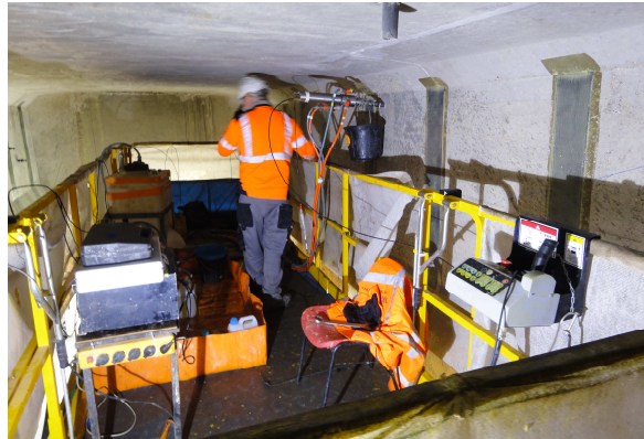
Figure 13: corrosion inhibitor impregnation workstation on platform
