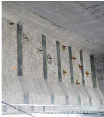
Figure 11 : injectors along the cables layout
