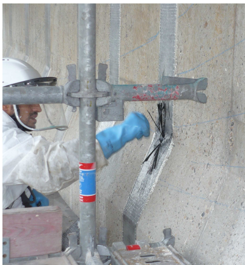
Figure 5: anchoring against pull-out forces in vertical strips.
