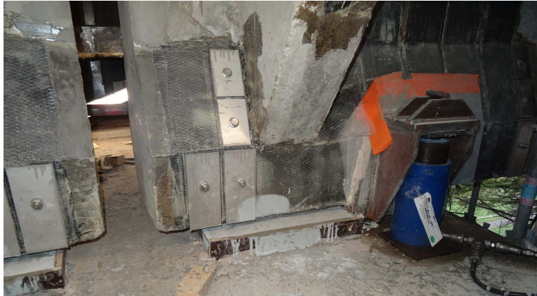
Figure 7: beam extremity: CFRP sheets anchorage with stainless steel plate
