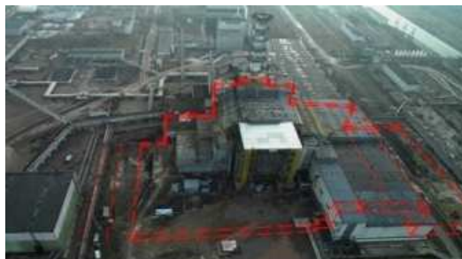
Figure 2: The damaged reactor, unit 4, and final position of the NSC shown in red
