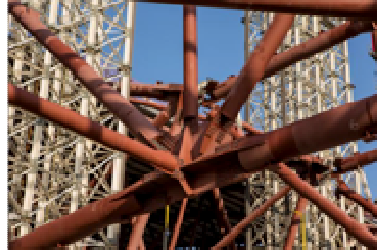
Figure 9c - connecting joints of the metal tubes
