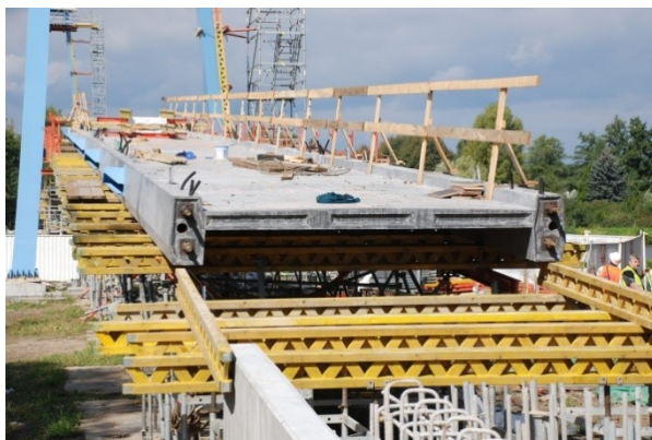
Fig. 11: Side span on the light scaffolding
