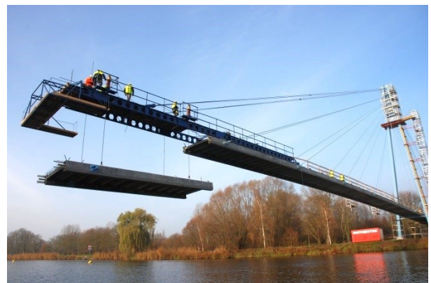
Fig. 12: Segment lifting by launching gantry
