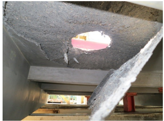
Figure 10: Punching of the slab
