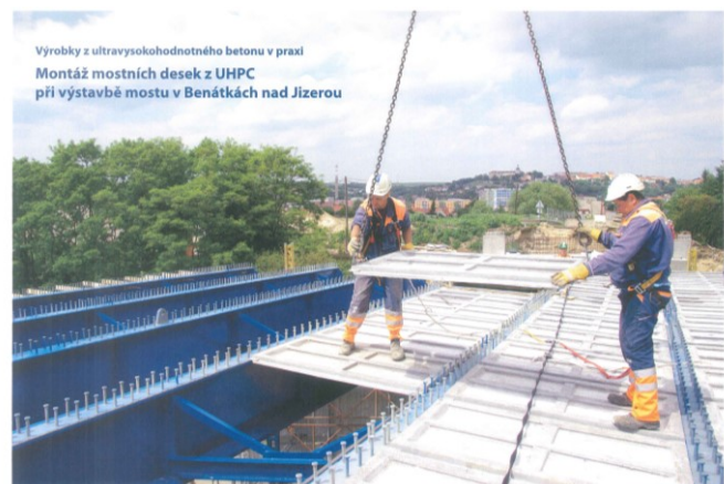
Fig. 4: Installation of UHPC permanent formwork
