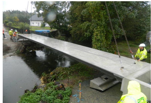
Fig. 3: Installation of the UHPC beam
