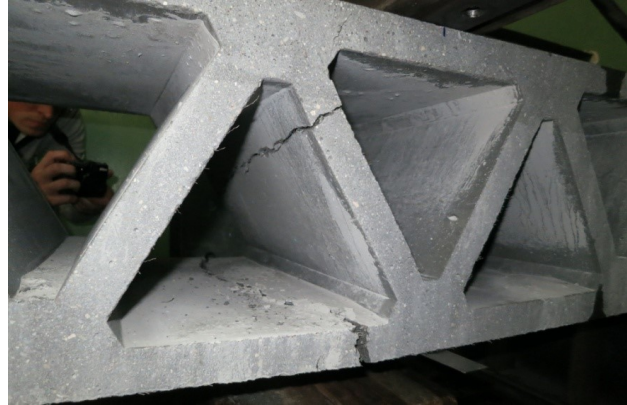
Figure 3: Main crack resulting in failure of the slab
