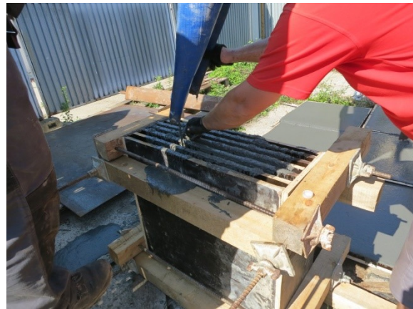
Figure 7: Casting in the vertical position
