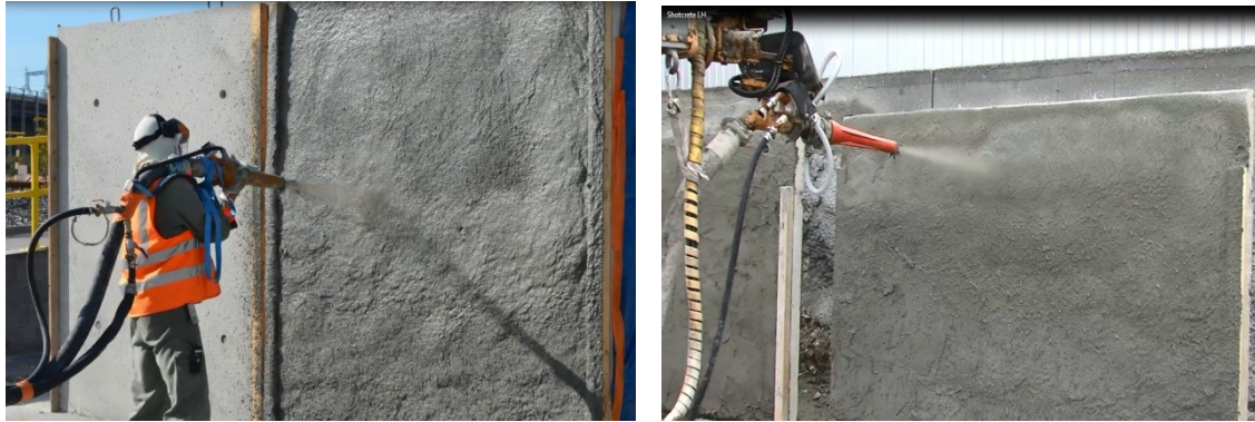
Figure 2a) Manual UHPC sprayed on a sandblasted concrete wall (60 mm thickness); 2b) UHPC sprayed by robot
