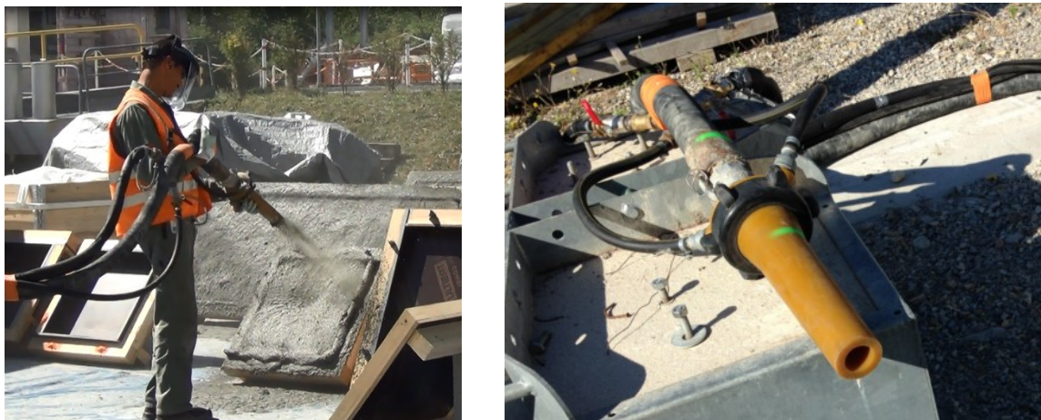
Figure 3a) Manual UHPC spraying in boxes for producing plates for mechanical and durability tests; 3b) Wet-mix nozzle with 45 mm exit diameter
