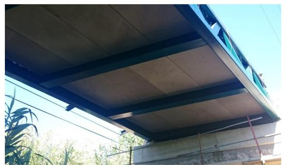
Figure 3: Inferior face view of the precast UHPFRC slabs of the bridge
