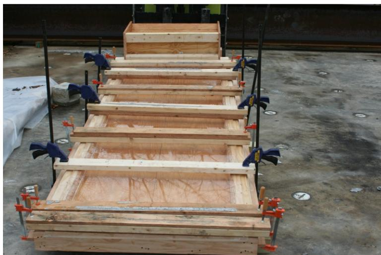
Figure 1. Formwork for casting of thin slab elements
