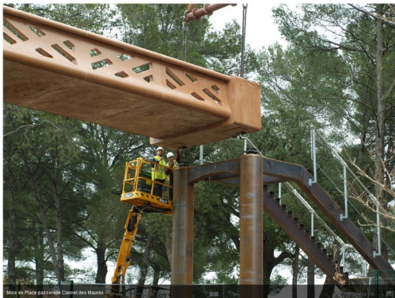
Figure 7: Placing the deck on its supports
