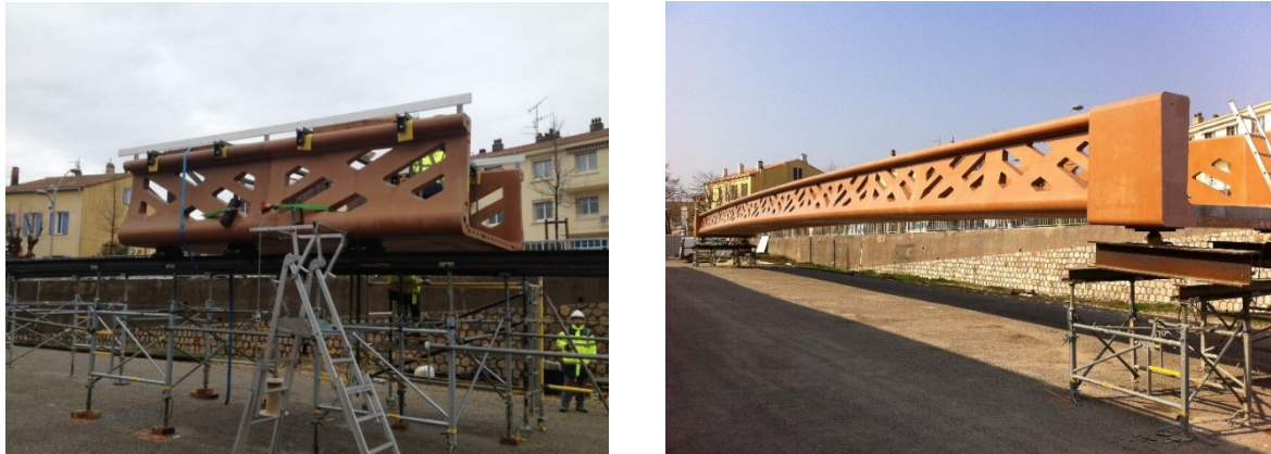
Figure 5: Placement of the first two segments on the temporary structure
