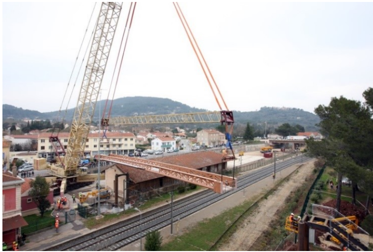
Figure 6: Lifting operation of the deck in a very constrained environment
