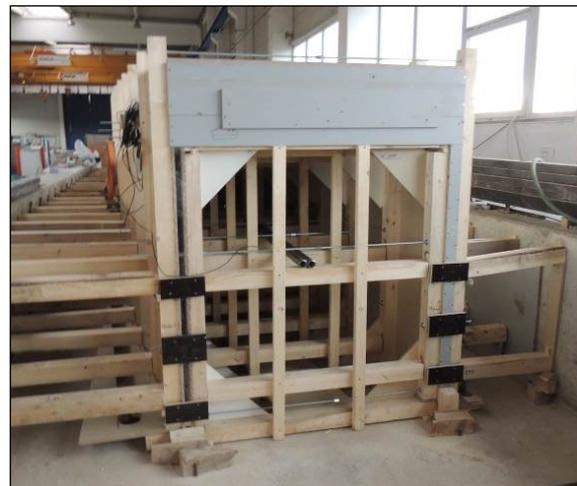
Figure 10: Formwork prepared for the casting
