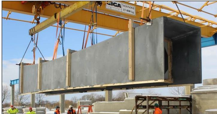
Figure 14: Transport of final footbridge in upside-down position
