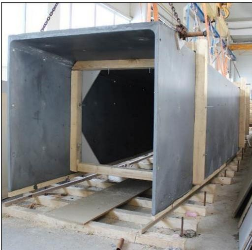
Figure 11: Demoulding of footbridge
