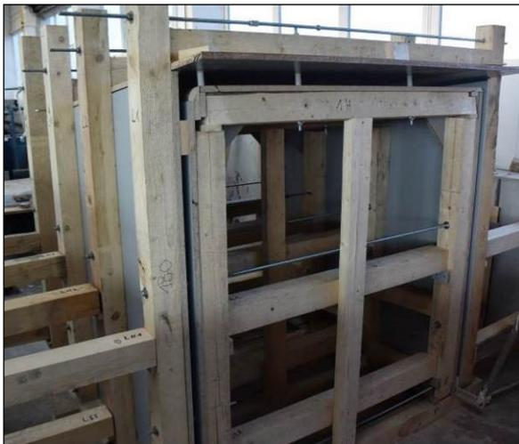
Figure 3: Formwork of the preliminary mock-up
