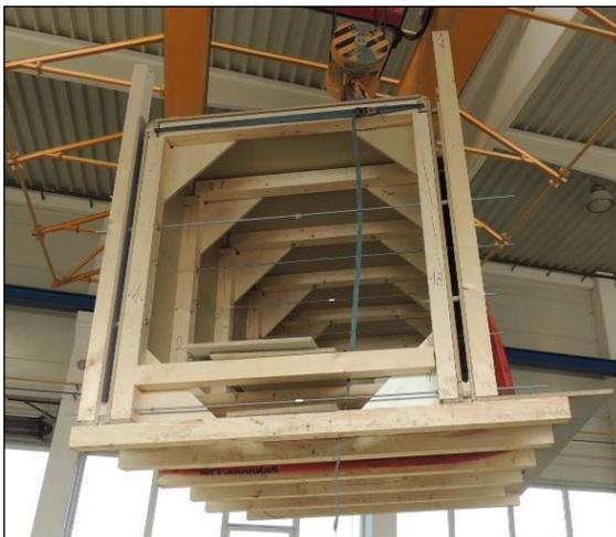
Figure 9: Transport of the ¼ of the formwork
