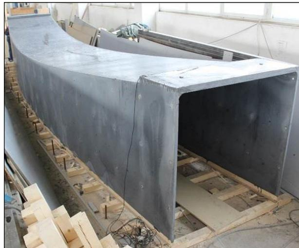
Figure 12: Final footbridge after demoulding
