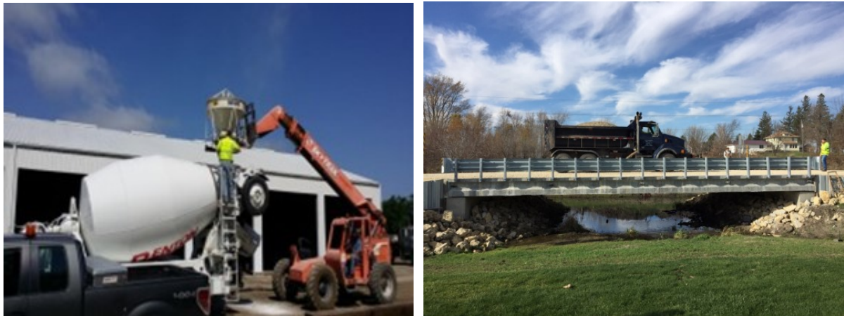
Figure 5: Ready-mix truck for the fabrication of UHPC girders and view of the completed bridge
