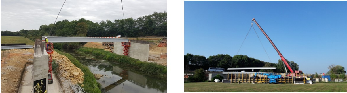
Figure 9: Installing the beams
