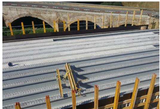
Figure 10b: Installing the precast panels
