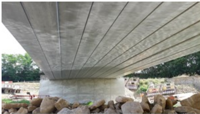
Figure 10a: bridge soffit
