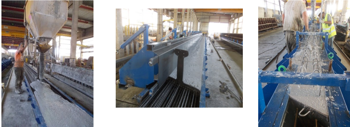
Figure 7: Concreting the beams
