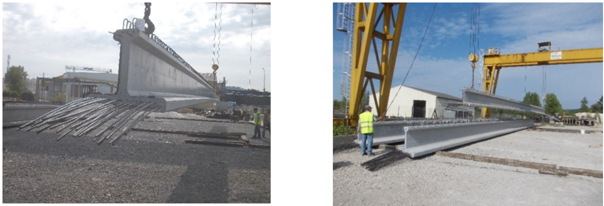
Figure 8: Beam transfer and storage
