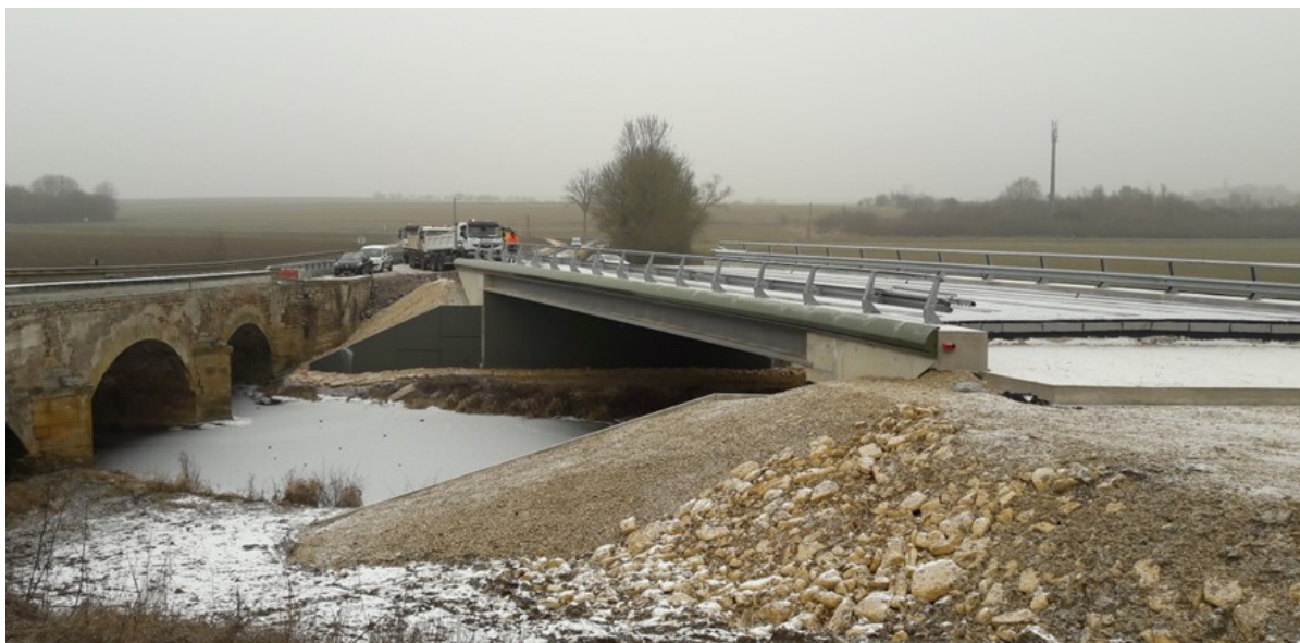
Figure 1: Overview of the structure (old and new bridges)
