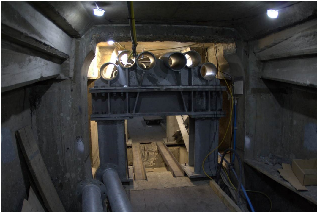
Figure 9: Long tendons deviator installation
