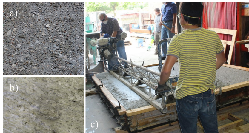
Figure 5: UHPC overlay trial in the laboratory: a) surface with exposed aggregates; b) broom-finished surface; c) placing of UHPC on one of the slabs
