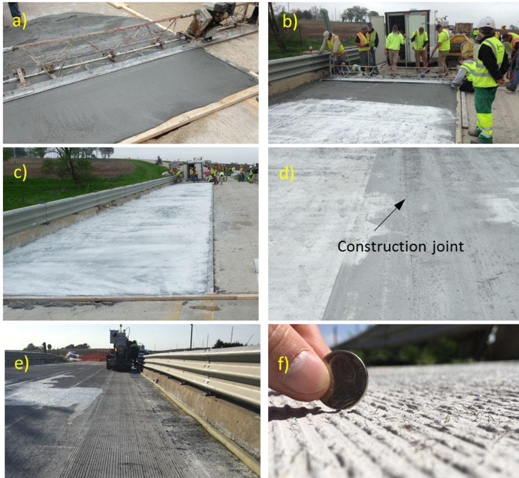
Figure 7: UHPC overlay on Mud Creek bridge deck: a) trial run; b) placing of UHPC on the deck surface; c) Lane 1 after placing UHPC; d) construction joint after grinding part of the deck; e) grooving of the surface; f) finished surface
