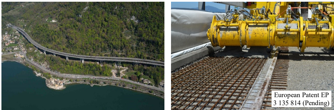
Figure 2: Chillon Viaducts and placing of UHPC on bridge deck
