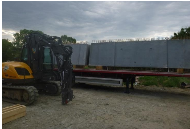
Figure 5: Delivery of the slabs to the construction site
