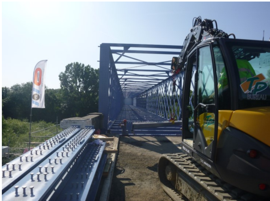
Figure 6: Installation of the reformed and welded sections
