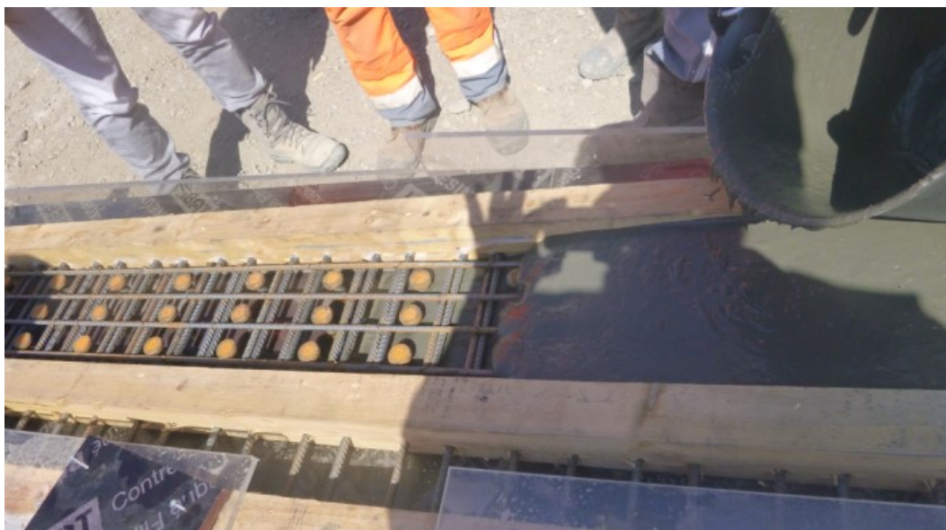
Figure 4: First test of field cast UHPFRC connection
