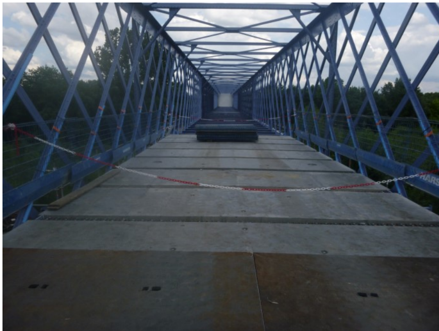
Figure 8: Slabs in place
