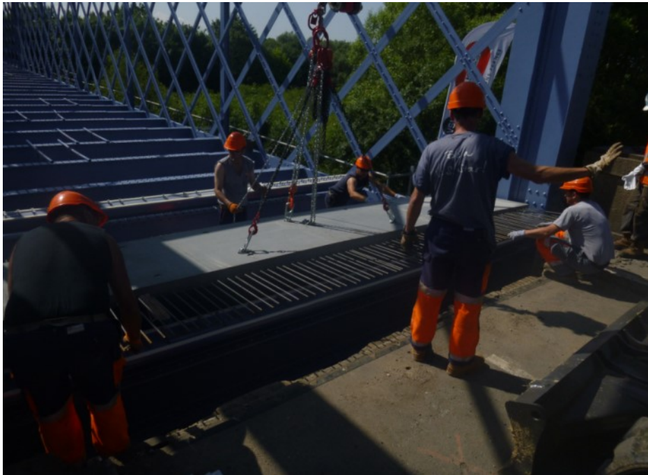
Figure 7: Laying the first slab
