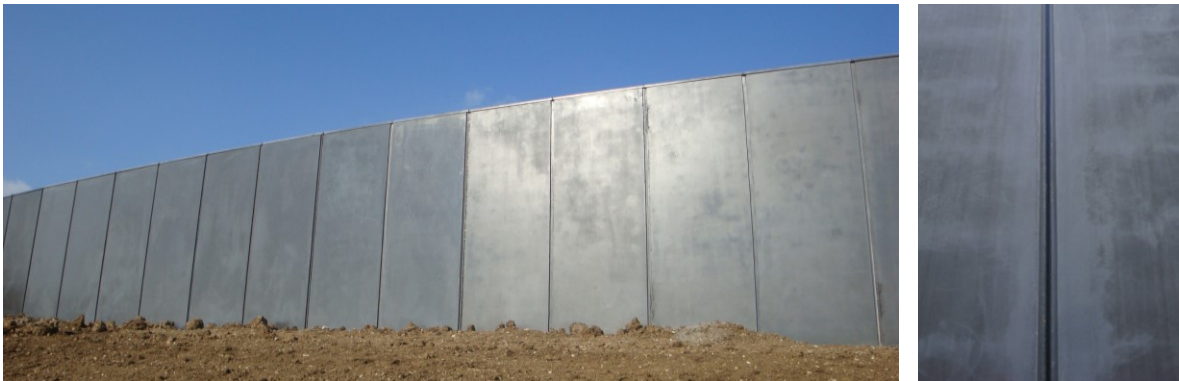
Figure 10: View of the limit between the reinforced segments and the normal one, four kinds of joints with only one aspect (left) PVC profile in the joint (right) (Pictures R. Fabbri)
