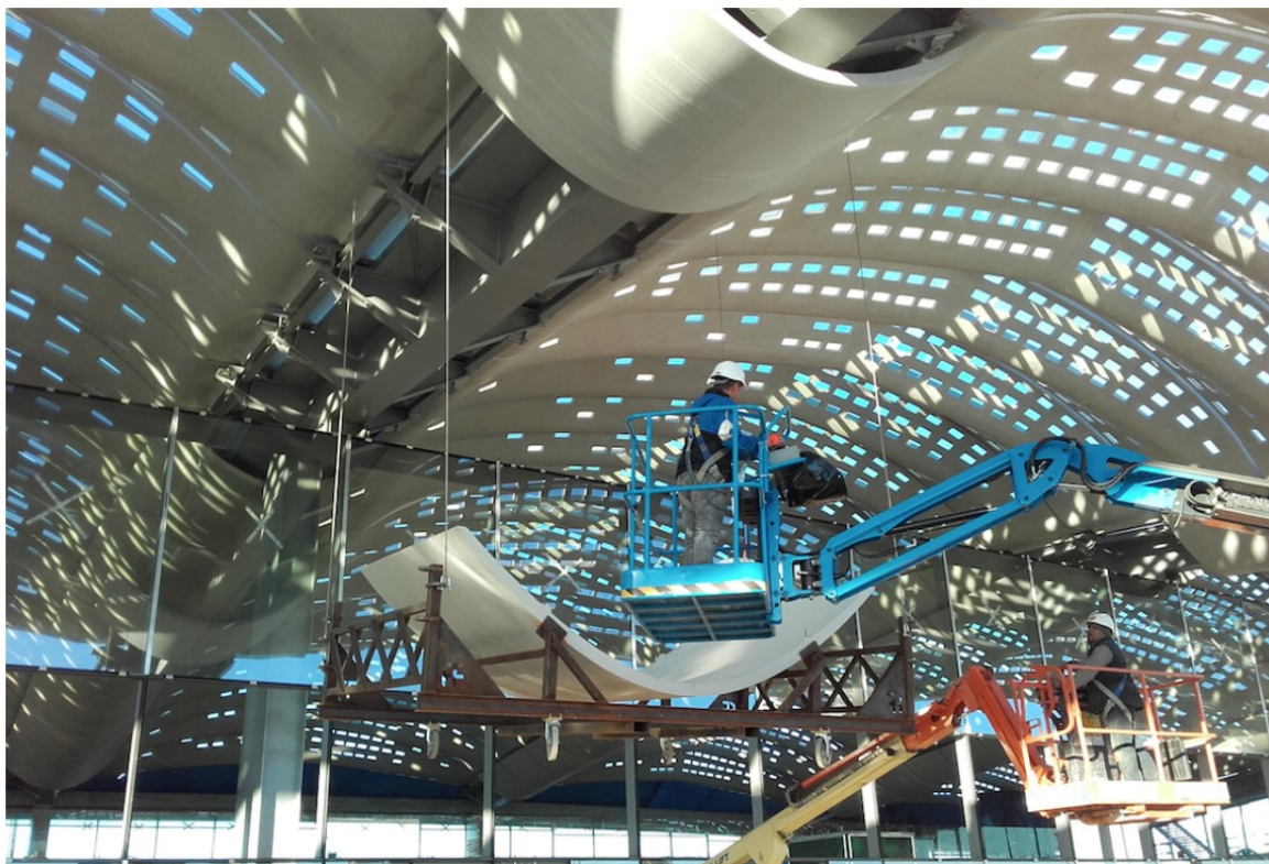
Figure 30 – Installation of shells with the aid of a cradle
