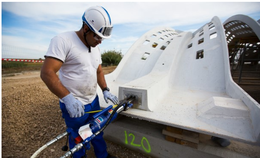
Figure 26 – Post-tensioning
