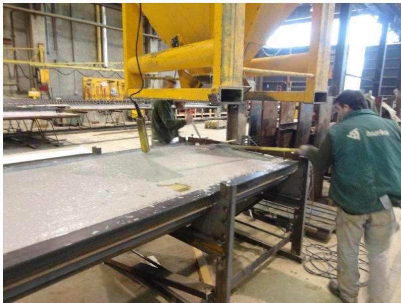
Figure 8: Casting the prototype in the prefabrication factory
