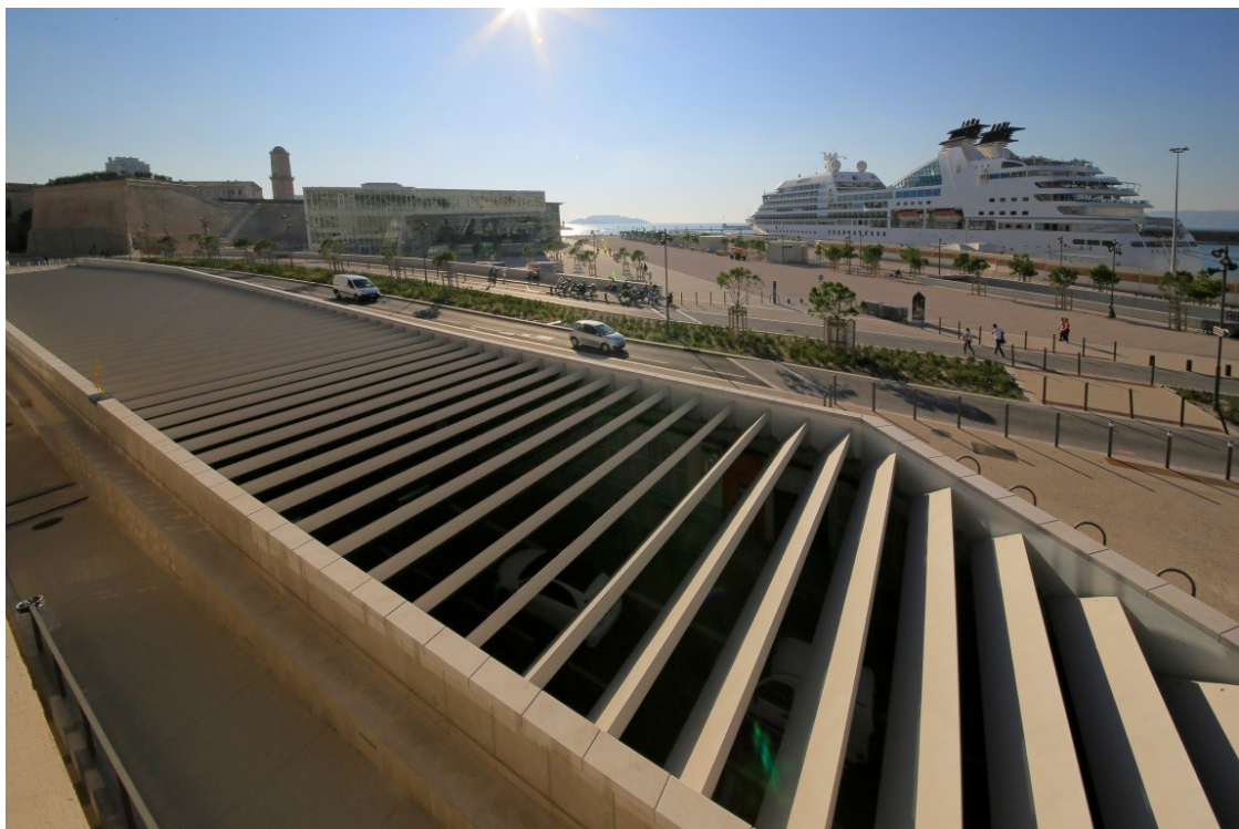
Figure 12: Global view after completion
