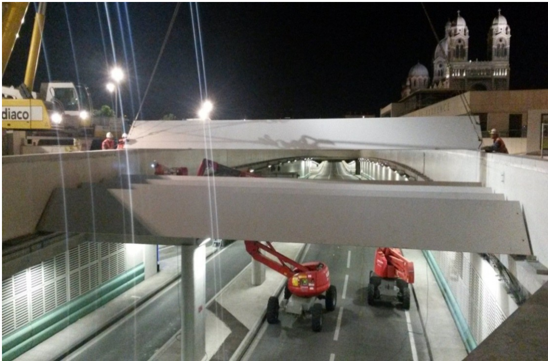
Figure 11: Nightly installation of the sunshades, using a 70T mobile crane
